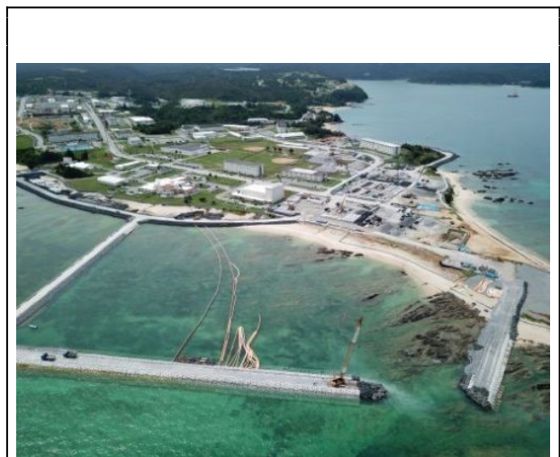
Sea Wall Construction at Henoko, Ryukyu shimpo , 19 July 2018.
