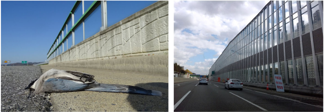
Figure 1. Examples of roadside noise barriers in the Republic of Korea. Left: an example of a transparent noise barrier with a collided Azure-winged Magpie Cyanopica cyanus ; right: a partially transparent noise barrier that is >2 km in length.
