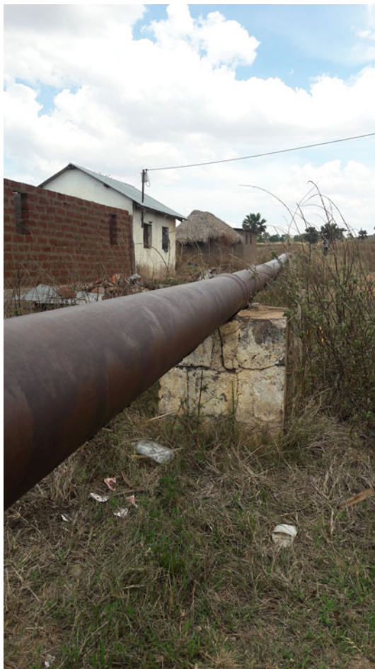
Figure 3. Rewelded pipeline between the pump station and the irrigation site.
