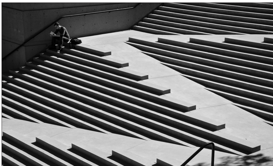
Figure 3. A visual representation of universal physical access in this photo of the blended ramp and steps at Vancouver, British Columbia's Robson Square, designed by Canadian architect Arthur C. Erickson in 1980.
