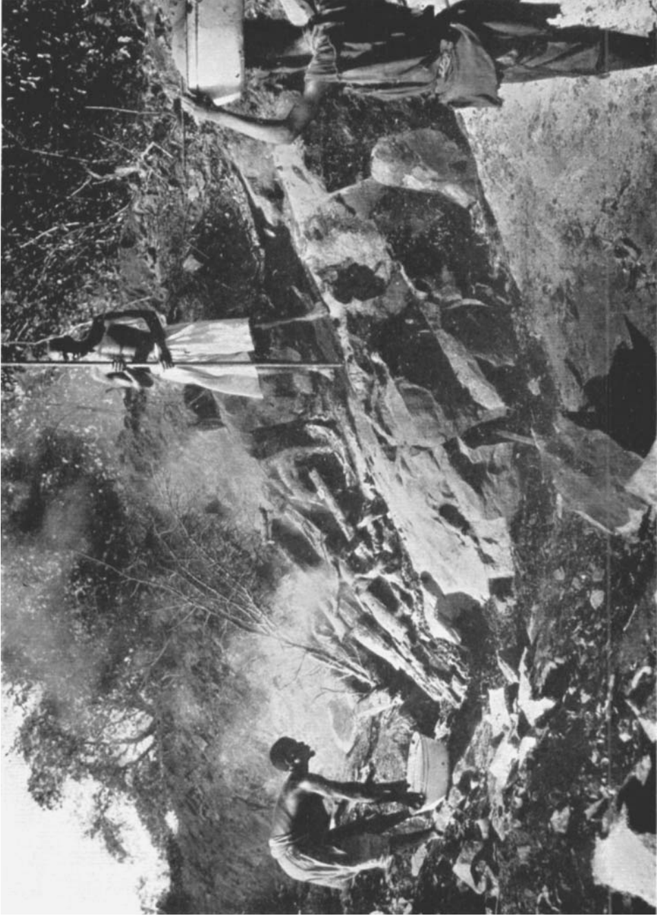
Fig. 13. NATIVES OF FRENCH GUINEA DESTROYING ROCKS BY THE FIRE-AND-WATER PROCESS DURING ROAD-CONSTRUCTION. (See p. 426) Ph. Euze de Chételet, 1932
