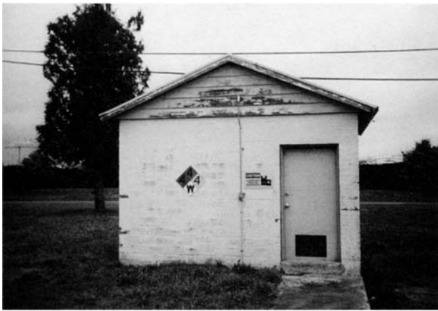
Figure 2. Hazardous Waste Disposal Building that previously contained unlabeled and improperly stored hazardous waste, North Pacific Division Laboratory, Troutdale, Oregon.
