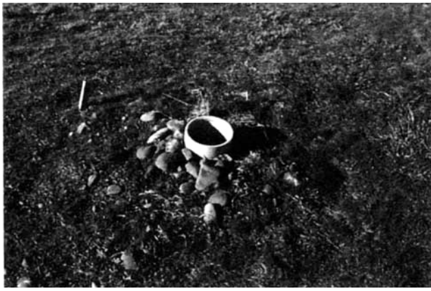
Figure 6. Hazardous waste disposal well, North Pacific Division Laboratory, Troutdale, Oregon.
