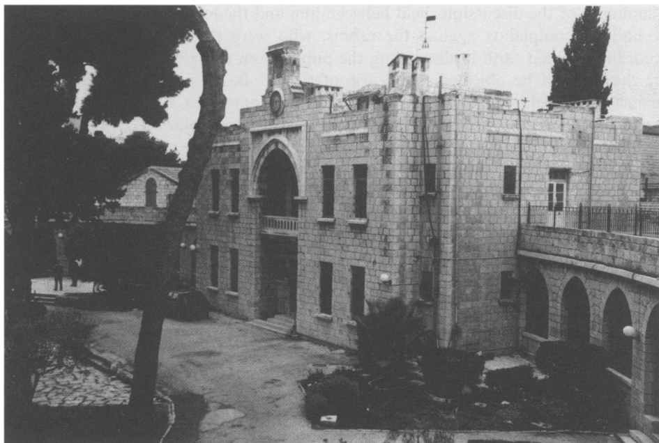
Figure 3: The former hospital in Jerusalem as it is today. It is now houses a school run by the Church Ministry among the Jewish People (originally the London Jews' Society). (Photo: Yaron Perry, 2001.)
