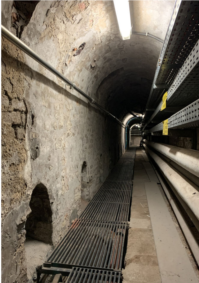
Figure 7. Filarete. Ospedale Maggiore, male ward, subterranean sewer corridor, lower canal underneath metal grating at bottom, upper canal through arched openings at lower left, large openings of latrine drains and small openings of ventilation pipes alternating on vault above, 1456–76, Milan. Author's photo.
