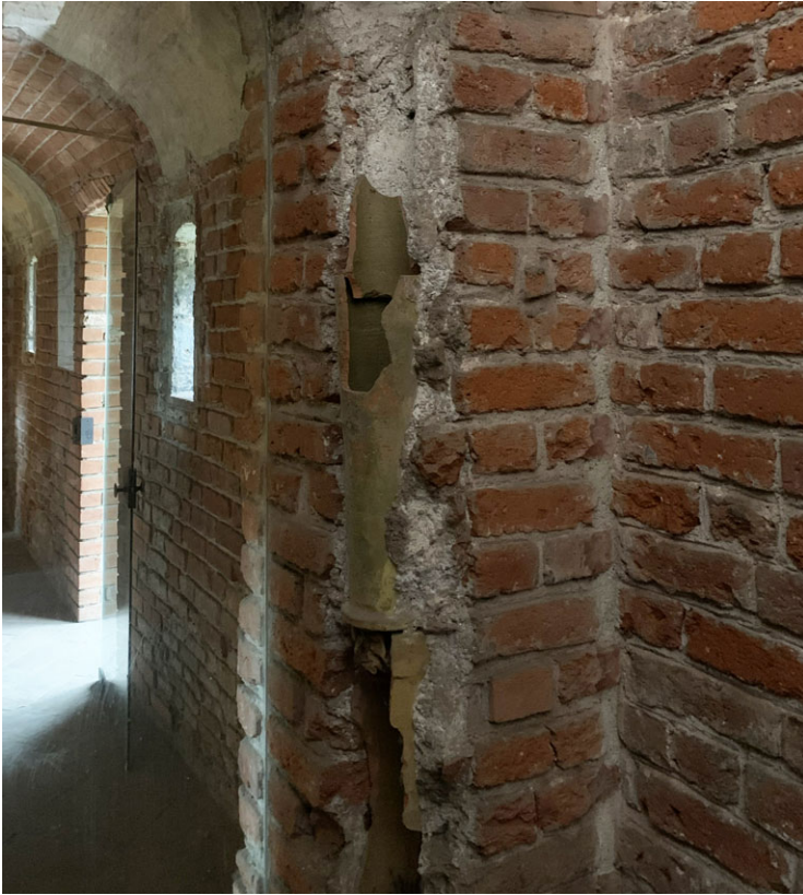
Figure 14. Filarete. Ospedale Maggiore, male ward, exposed terracotta ventilation pipe, 1456–76, Milan. Author's photo.
