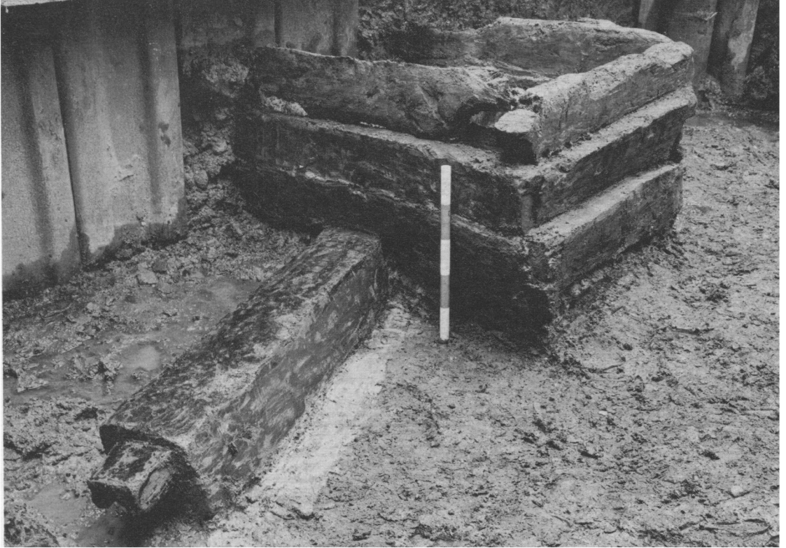
A. London: a timber-lined water-tank and wooden pipe, pierced at top and bottom; Lower Thames St. (p. 268).
