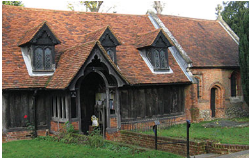
St Andrew's Church at Greensted in Essex, showing the eleven century timber walling of the nave. Photograph: Judith Roberts.
