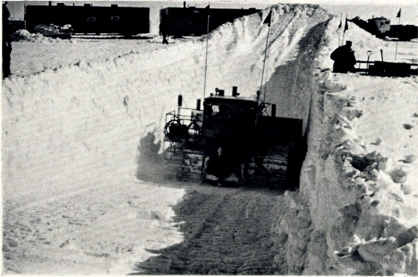
Fig. 4. Excavating a pit
