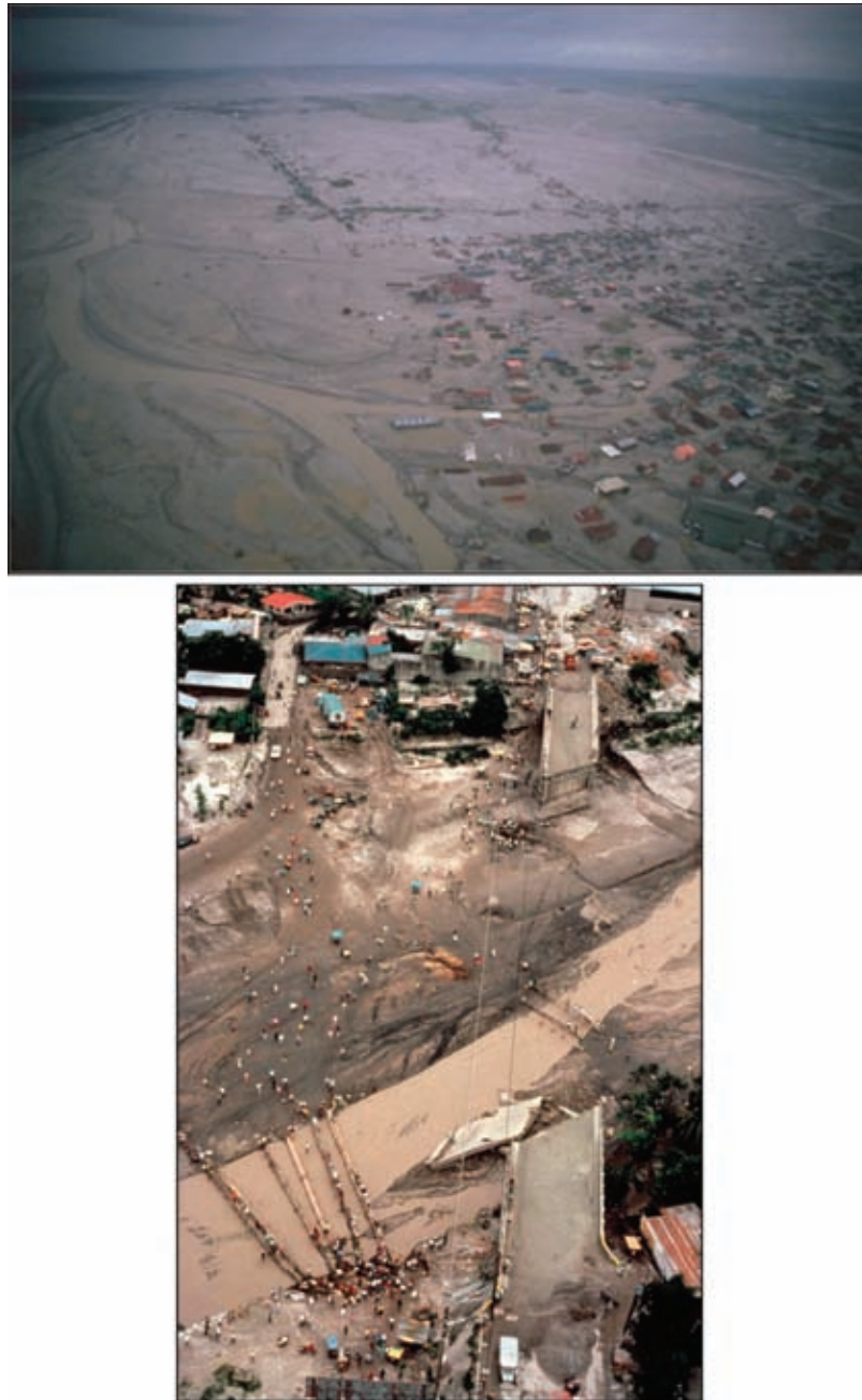
Figure 1.5 a) Only the roofs of 2-storey buildings are visible after repeated inundation by lahars following the 1991 eruption of Pinatubo, Philippines (C. Newhall). b) Lahars during the 1991 eruption of Pinatubo in the Philippines caused the destruction of concrete bridges (USGS archive).
