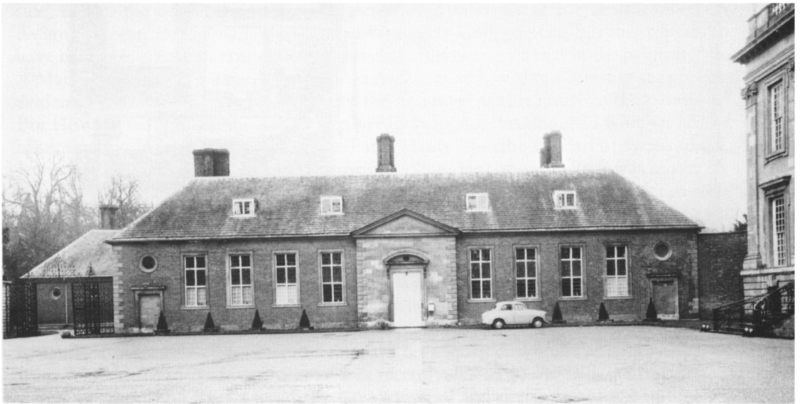
Fig. 17 Easton Neston. Kitchen, looking south
