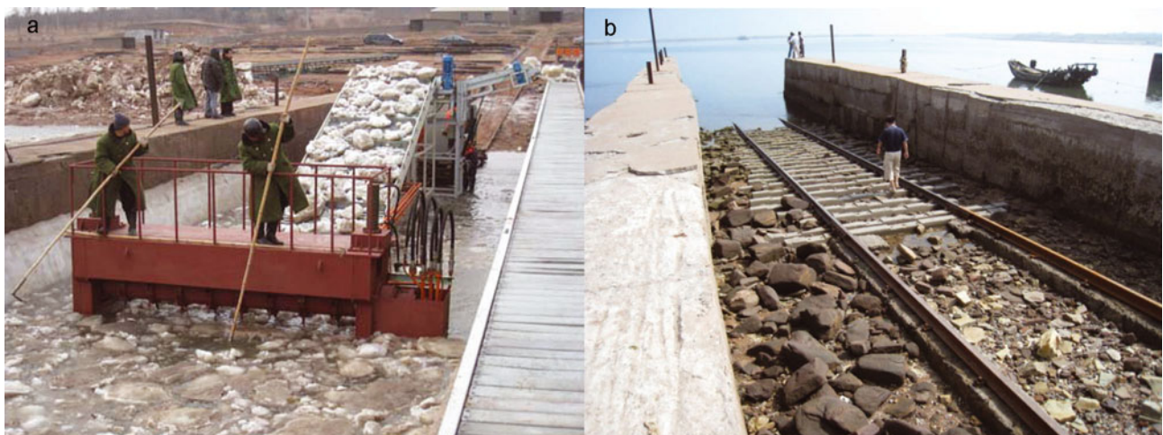
Fig. 2. Mechanical equipment for taking (a) sea ice and (b) ancillary facilities for ice mining with the shore-based technology.
