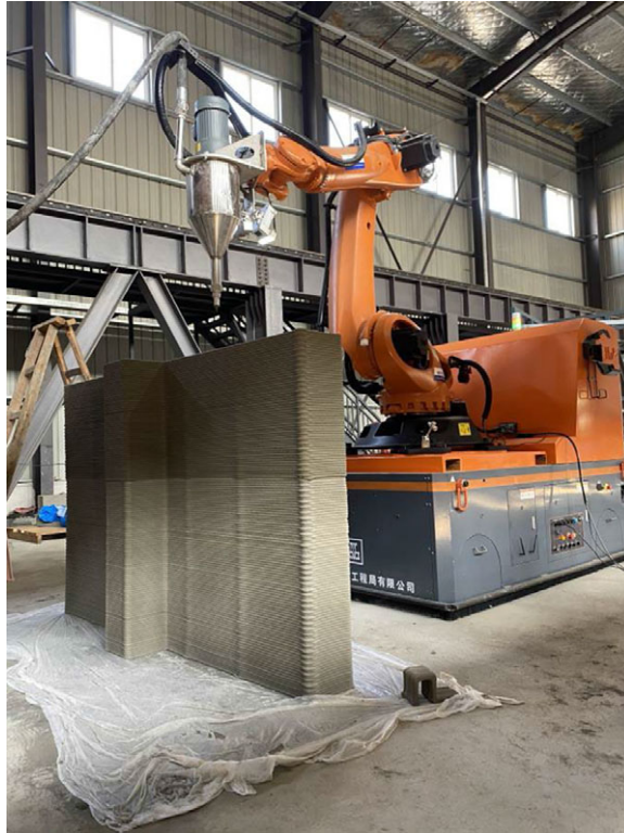
Figure 8. Concrete 3D printing with mobile manipulator for intelligent construction.
