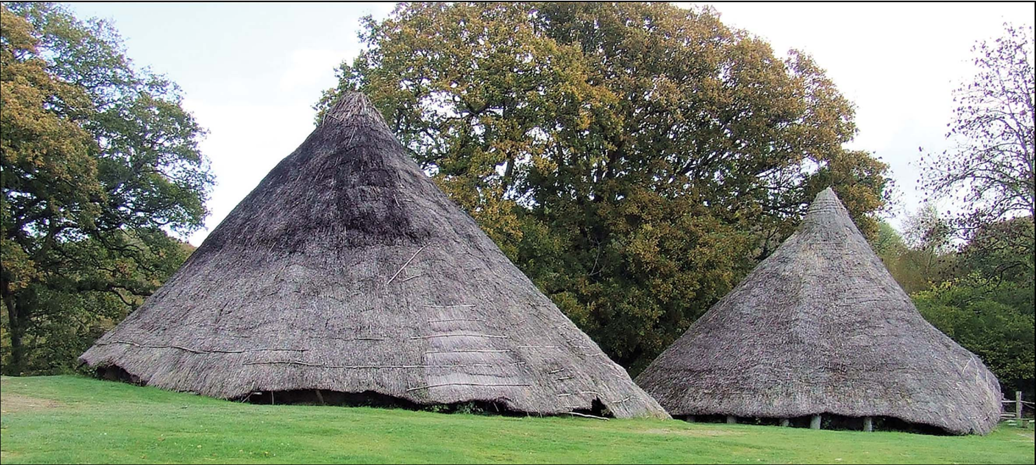
Figure 1. View of the Cookhouse (right) and the Earthwatch roundhouse (left) prior to their dismantling and excavation (photograph by H. Mytum).
