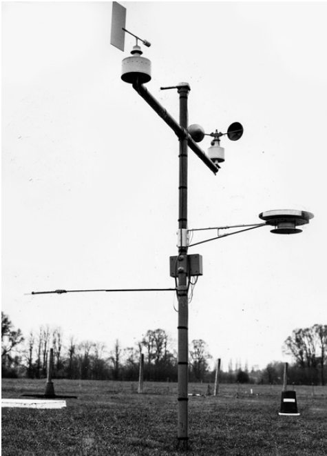
Figure 1.8 An early prototype automatic weather station at the then Institute of Hydrology in Wallingford, England, in the late 1960s. (Photograph by Ian Strangeways)
