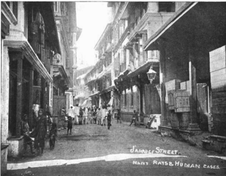
Bombay City: showing go downs on ground floor.
