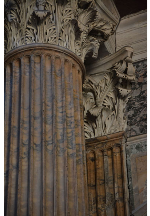
FIG. 39. Pantheon, rear apse, right side. Detail of upper fluting of free-standing columns. ( Photo: author )
