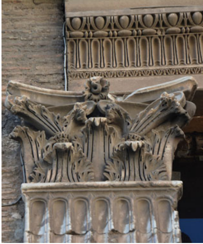
FIG. 40. Rome, Lateran Baptistery. Re-used pilaster from exterior entrance, upper fluting. (Photo: author)
