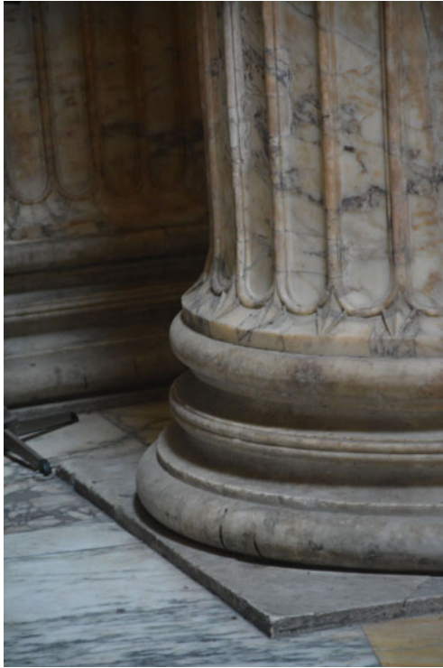
FIG. 38. Pantheon, rear apse, right side. Detail of lower fluting of free-standing columns and pilasters. ( Photo: author )
