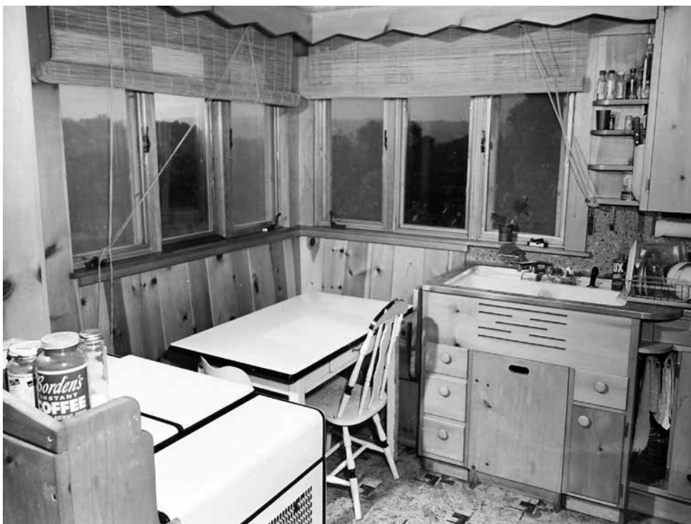
10 Mrs Galford's kitchen after the remodelling. The completed project included few deviations from the final plan [9]: moving the table from the middle of the room to the room's corner below the widows, shifting the stove from its location along the wall to the place occupied by the table on the plan, and forgoing the counter below the widows. Dept. of Household Economics and Management Research Studies, Division of Rare and Manuscript Collections, Cornell University Library #23-18-1648, Box 6.
