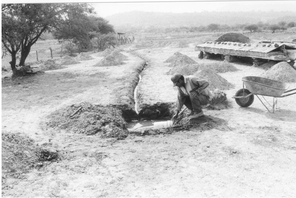
Figure 4. At Simirao there is a network of canals linking nearby springs to the saltworks. A constant flow of mineral-rich water from the thermal springs is essential for salt production. Photograph by the author.
