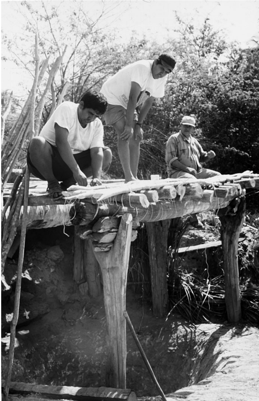
Figure 7. Building a tapeixtle to filter salty water was a laborious process involving several men. Photograph by the author.
