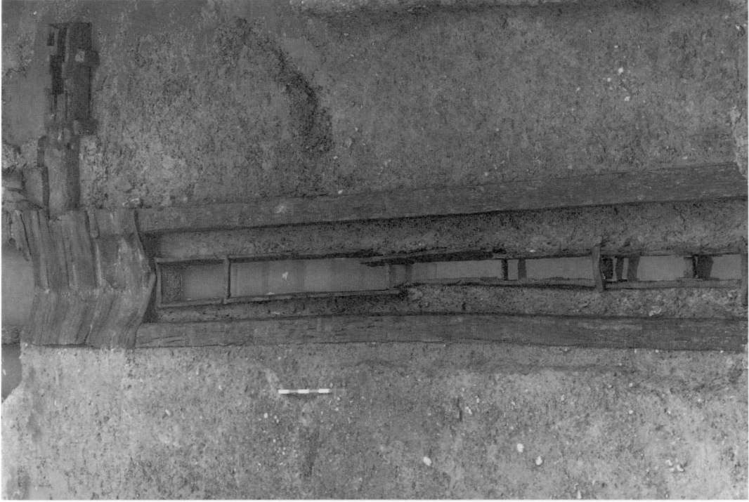
B. London: the main axial drain with the plank lid partially removed. (p. 59)
