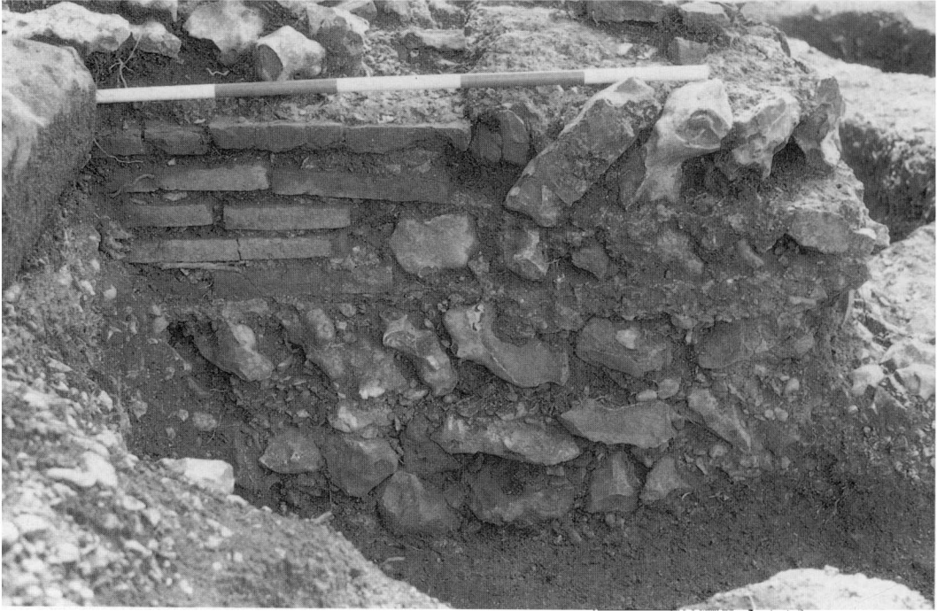
A. Silchester: the North Gate 1991: northern elevation of eastern footing of the gate. (p. 97) (Photo: M. Fulford)
