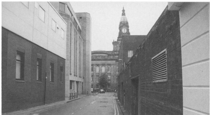
Fig. 14. Service areas for the precinct are bleak (Photo: author, 2012)
