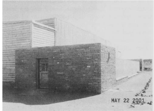
Figure 4. The Zuni eagle sanctuary from the west side, showing details of hand-worked native sandstone, stick latillas on the door, and lumber milled from the Zuni sawmill. The overall architecture incorporates the "blocky" multi-layered construction found in Zuni and other New Mexico Pueblos.
