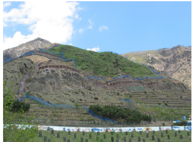
FIG. 5: Experimental reforestation at Ashio: The green zone at the top is a mix of soil, seed and fertilizer sprayed onto the rock in an attempt to compensate for the lack of topsoil. (Photo: Robert Stolz, 2002.)
