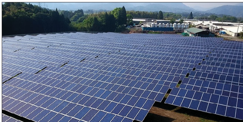
Photovoltaic power plant at Miyazaki Prefecture in Japan. Credit: Shizen Energy Inc.
