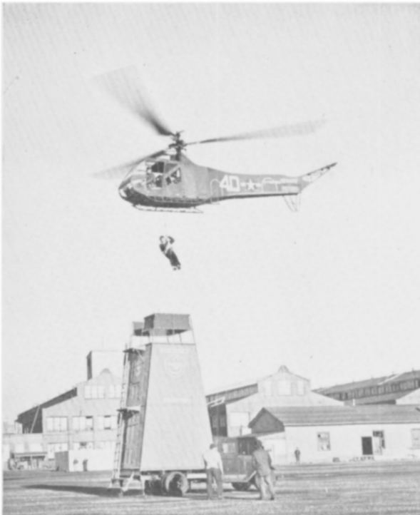
Fig. 4. Sikorsky R-4 helicopter—less conventional undercarriage—hovers well clear of ground cushion effect.
