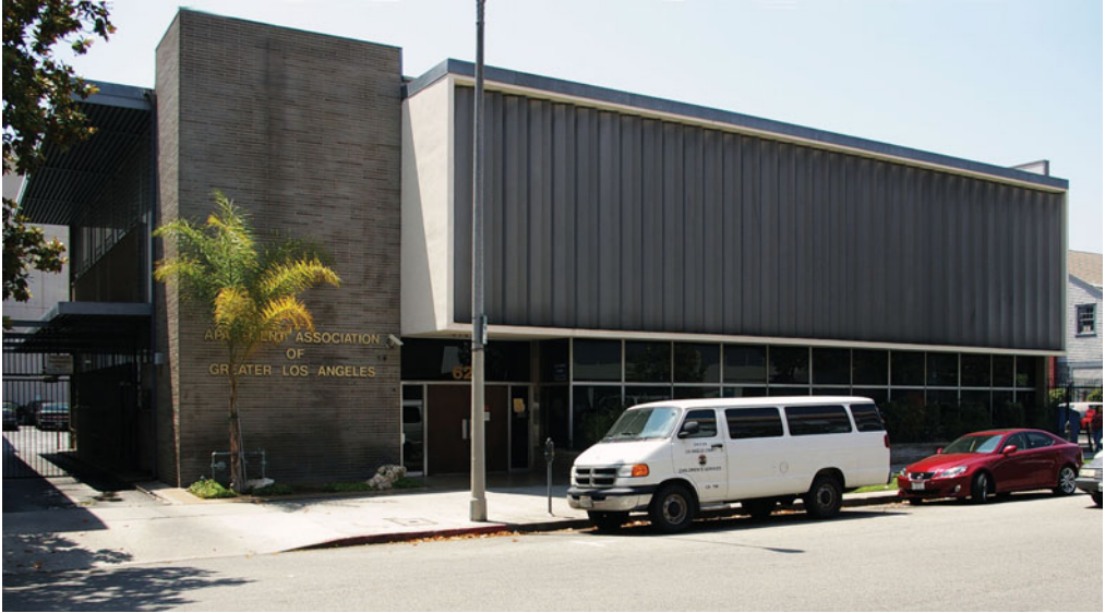
Fig. 14. Los Angeles, Richard Neutra's Northwestern Mutual Fire Association, showing sun-shading devices (author's photograph, 2009)
