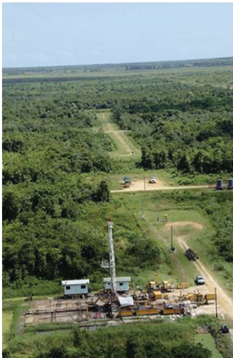
Fig. 13. A typical land location in the Tambaredjo Field. The swamp areas are poldered and drained prior to building the locations.
