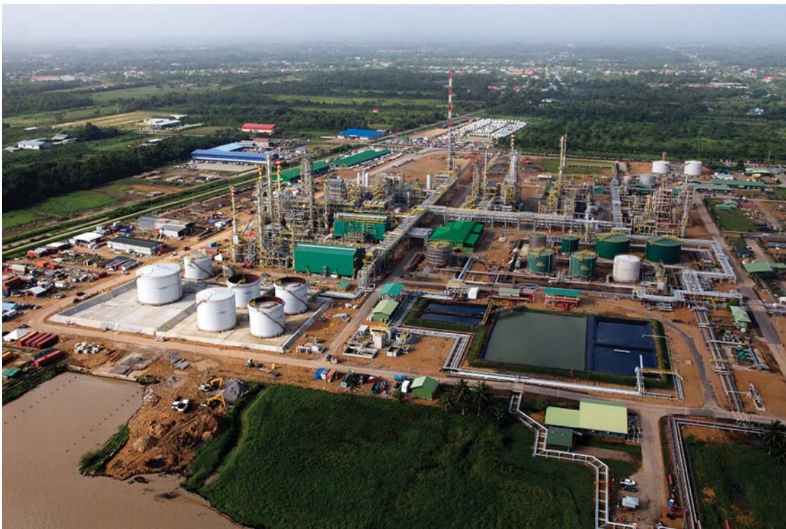
Fig. 17. View of the new Staatsolie Refinery taken from the Suriname River.
