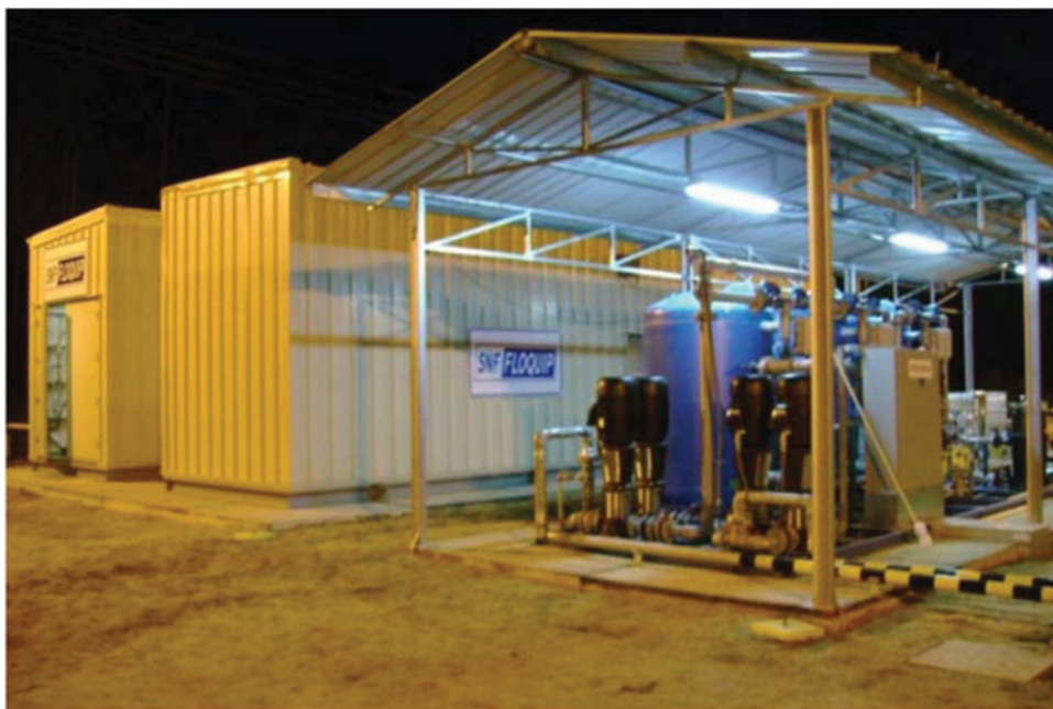
Fig. 15. Polymer Pilot Injection Plant at the Tambaredjo Field.
