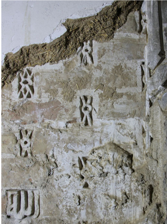
Fig. 9. Rising joint plugs to the left of the mihrab , including ones extending underneath the stucco corner columns.
