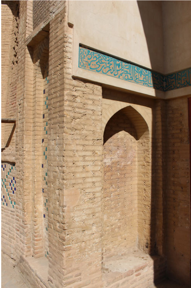
Fig. 18. Incised mortar bed patterns in brickwork on left side of the entrance to the mosque and the shrine in Natanz.
