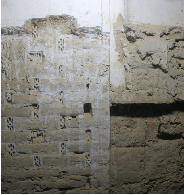
Fig. 7. Construction break beside the blind recess to the right of the mihrab , with the later engaged column extending down behind the (lost) lustre inscription band to the height of the top of the star and cross tile dado.
