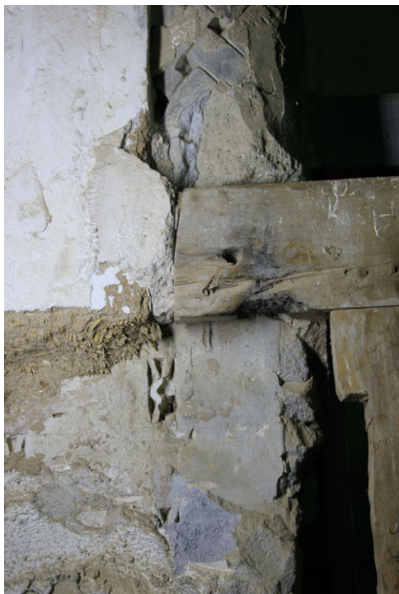
Fig. 6. Corner to the right of the mihrab recess; detail of the original brickwork and later column.
