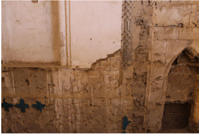
Fig. 4. Rising joint mortar decoration beneath the (lost) band of lustre tiles, 'Abd al-Samad Shrine, Natanz.
