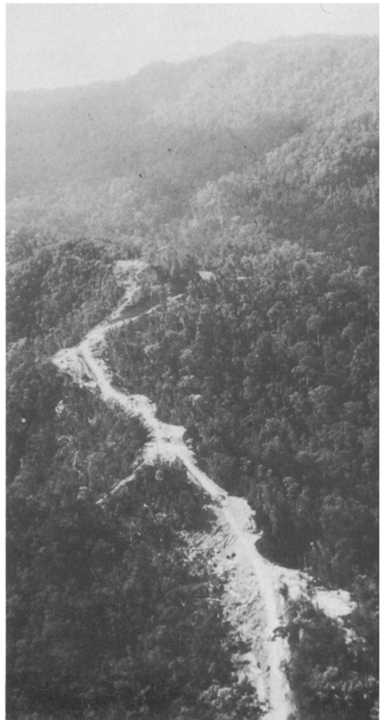
Ridgetop access road through part of the Sungai Tekam Concession (Andrew Johns).
