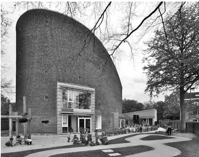
19 Kindergarten from the southwest with playground, showing new two storey bay that breaks through the old wall. The upper window is that seen in [16].
