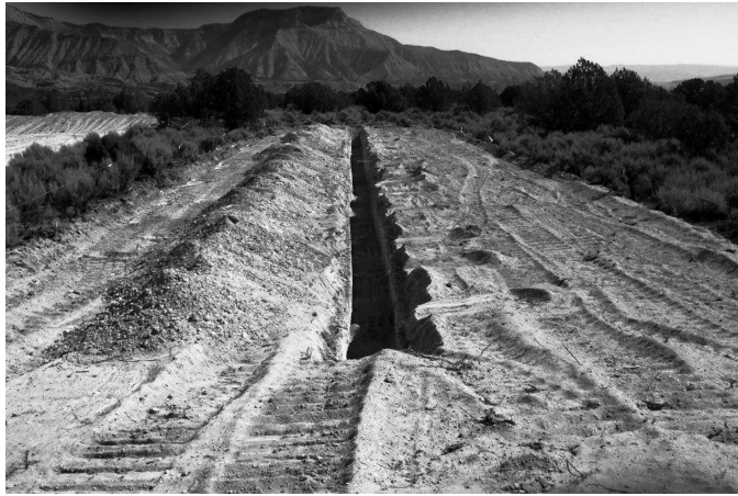
Figure 2. Pipeline disturbance simulation at the Grand Valley Mesa site.
