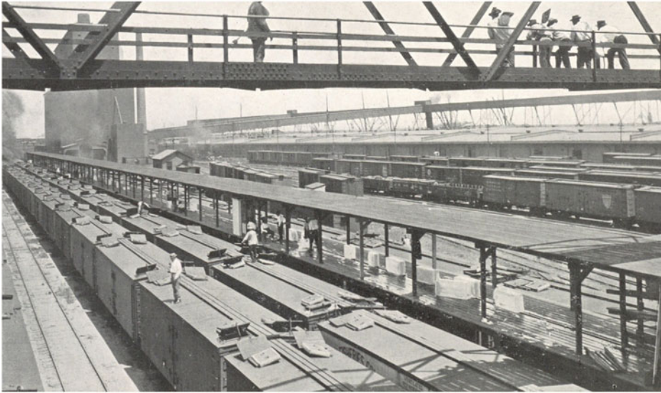
Figure 3. View of ice blocks and employees on so-called icing platforms in New Orleans. Each of these platforms could accommodate eighteen banana cars at once. “Icing Banana Cars at New Orleans, La.—An Important and Extensive Operation,” Fruit Dispatch 3, no. 4 (August 1917): 98.
