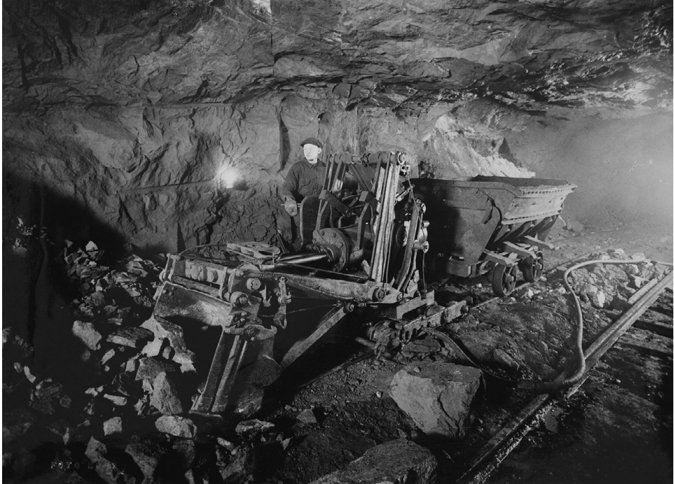
Figure 8.2 A loading machine in a mine. Photo: Foto Roos/Finnish Heritage Agency. CC BY 4.0
