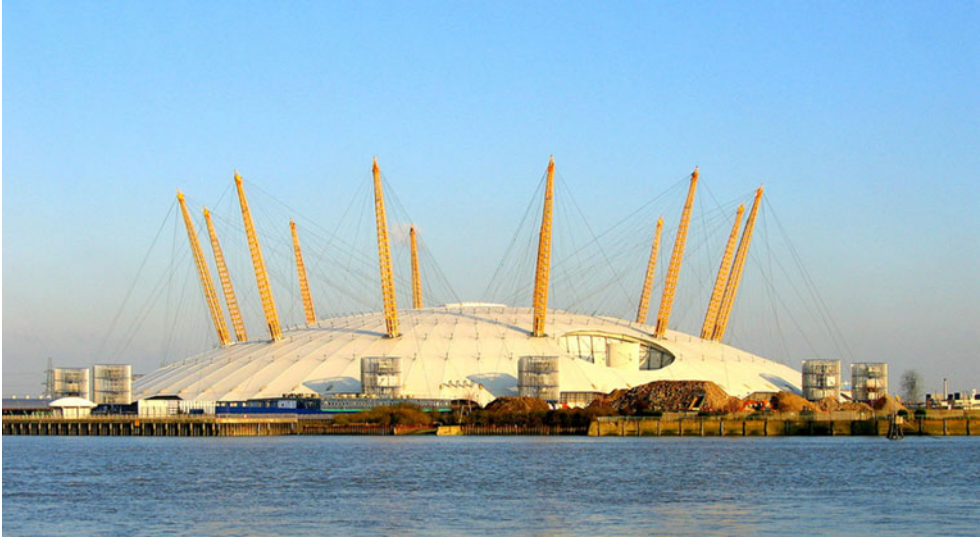
Figure 3. The Millennium Dome, Greenwich, UK. James Jin 2004, Creative Commons, www.flickr.com/photos/jamesjin .
