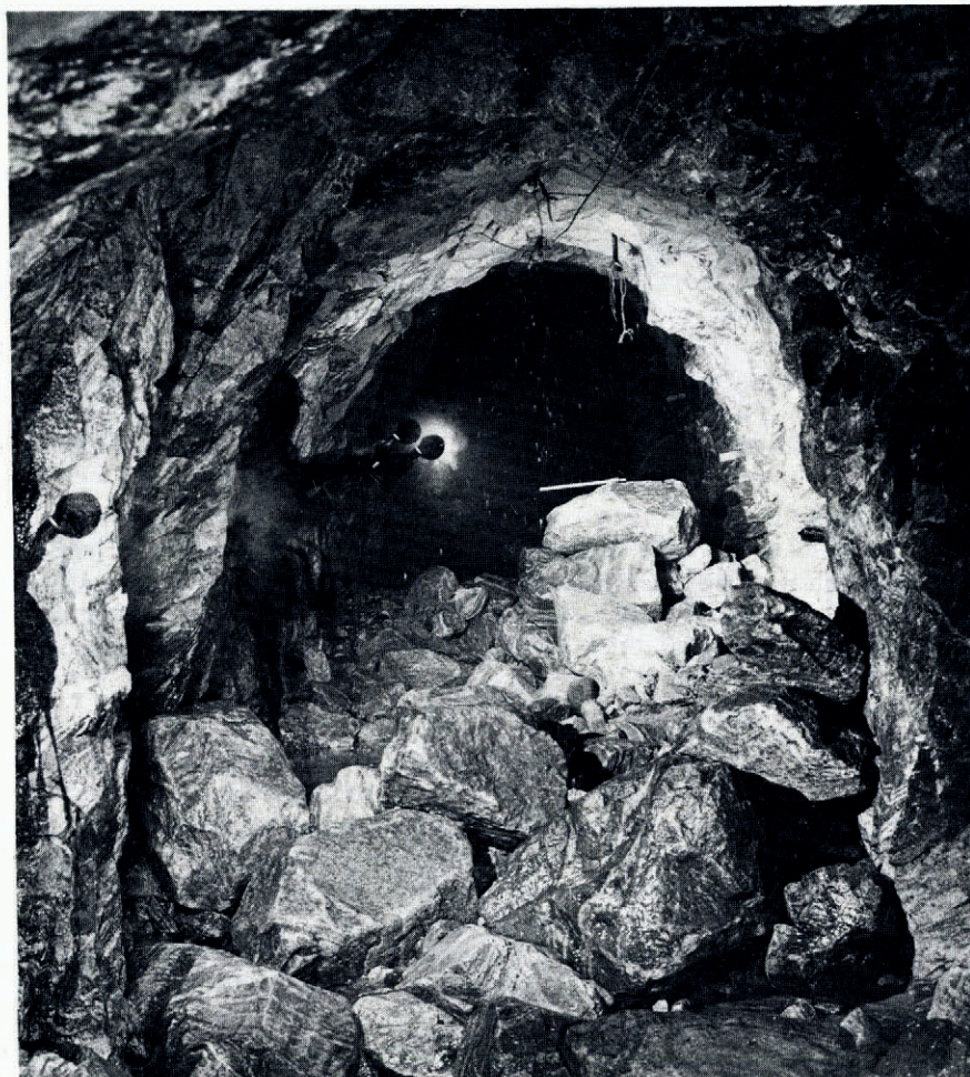
Fig. 5. Coarse material carried by melt water from a subglacial intake during the summer of 1974. Such material must not be allowed to enter the almost horizontal diversion tunnels (the galleries).
