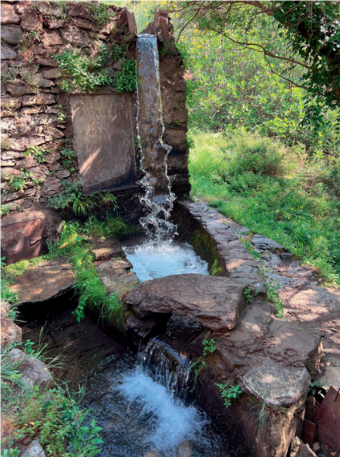
Figure 33 In the Alpujarra, as the surface canal rushing down from the mountain drops in level, a regulating basin slows its speed (photo: H. Varden)
