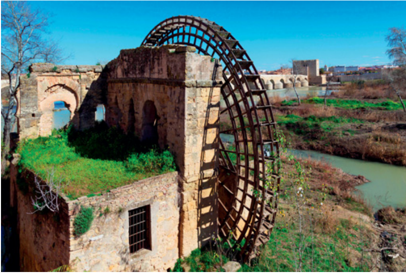
Figure 22 Aboulafia waterwheel and bridge at Cordoba (photo: Daniel Martín Trani/Alamy)
