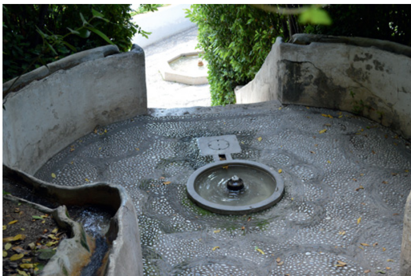
Figure 35 In the water stairway at the Generalife the water drops into the small depression on the lower left, slowing its flow (photo: D.F. Ruggles)
