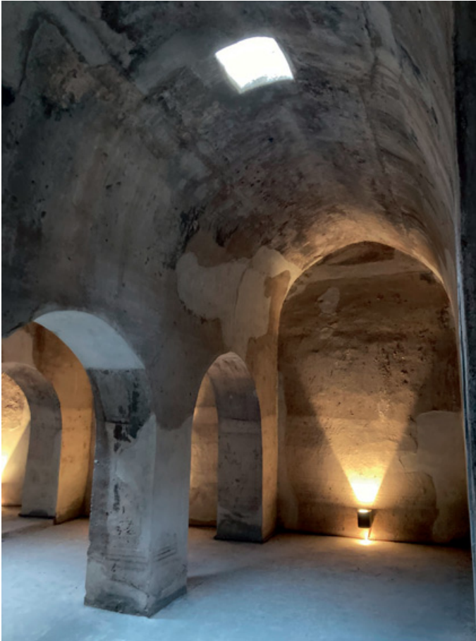
Figure 12 Barrel-vaulted interior of the Aljibe del Rey, Granada. Skylights allowed rainwater to enter the cistern during the rainy season (photo: D.F. Ruggles)
