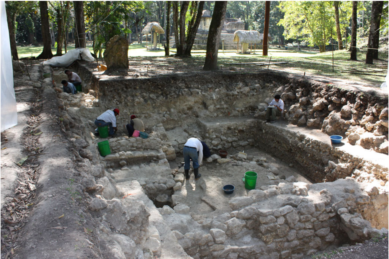
Figure 9. Extensive excavations of the A-24 Platform in Group A of Ceibal that revealed Structures Kelko, Ba'ba'y, Kotko, and Kaaxkuut and Platform Saq', dating to the Escoba phase. Photograph by Aoyama.
