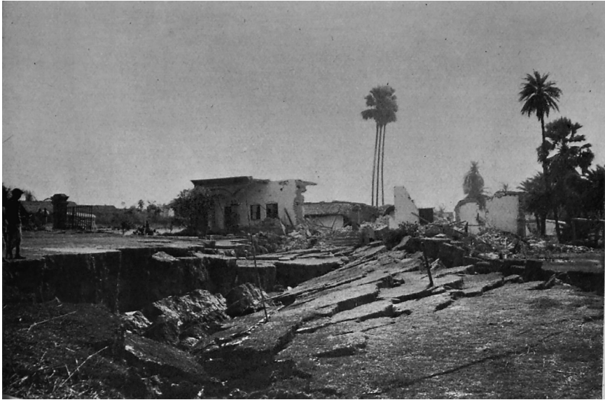
Image 2.3 Slumping of the ground along the lake in Motihari documented by the Geological Survey of India officer J. B. Auden.
