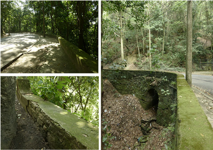
Figure 10. Remains of the Carioca Aqueduct Source: Photographs by the authors, 2014.
