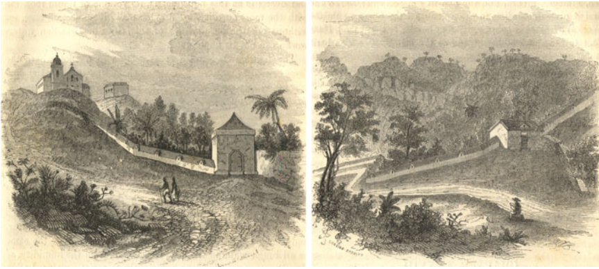
Figure 3. Aqueduct and caixas
