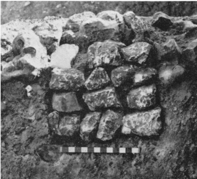
B. Chalk: Niche 3 before removal of blocking: scale in inches (p. 118).
