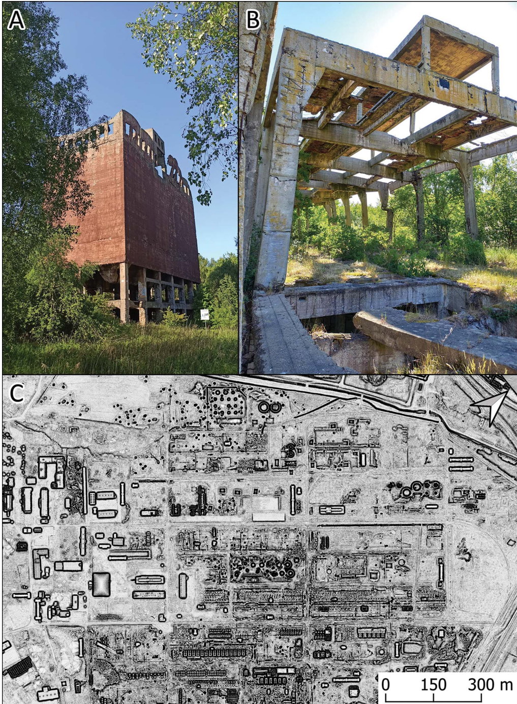
Figure 8. The ruins of the plant: A) the multi-storey coal mill; B) the concrete frame of the coal power plant; C) preserved relics of the plant registered by ALS (openness-positive) (figure by G. Kiarszys).
