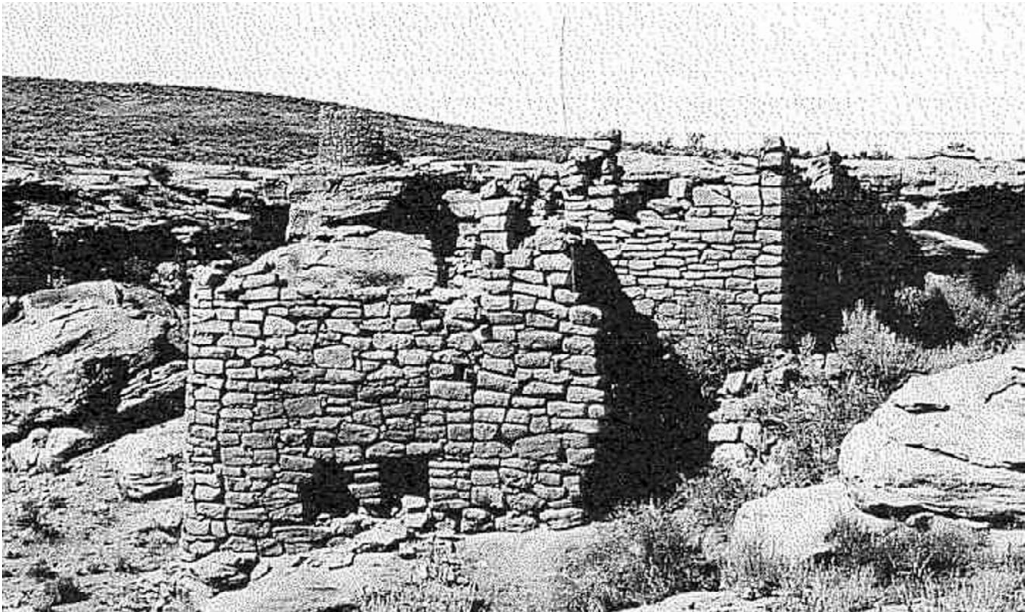
Figure 6. Unit-Type House, east room, east exterior. Courtesy Smithsonian Institute, MS4321
