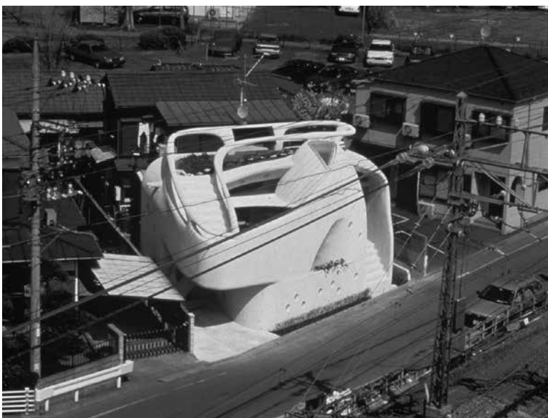
2a,b Truss Wall House, interior and exterior
