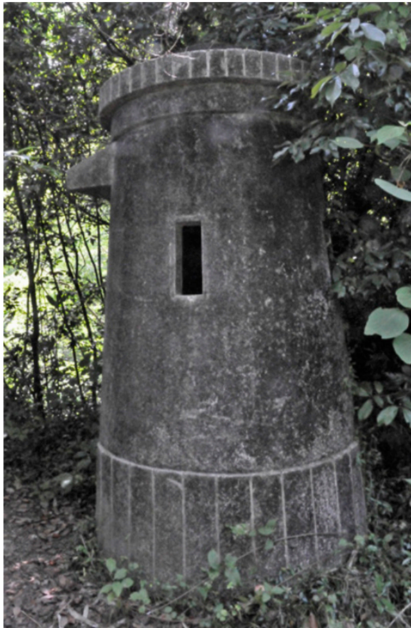
Military Tower on Ninoshima Island, on top of a bomb shelter and artillery storage hill, Japan, 2008
