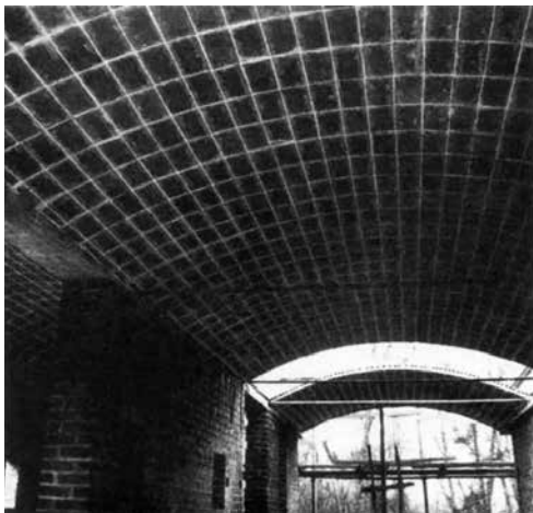
18 Xinzhai Coffee House, under construction.
