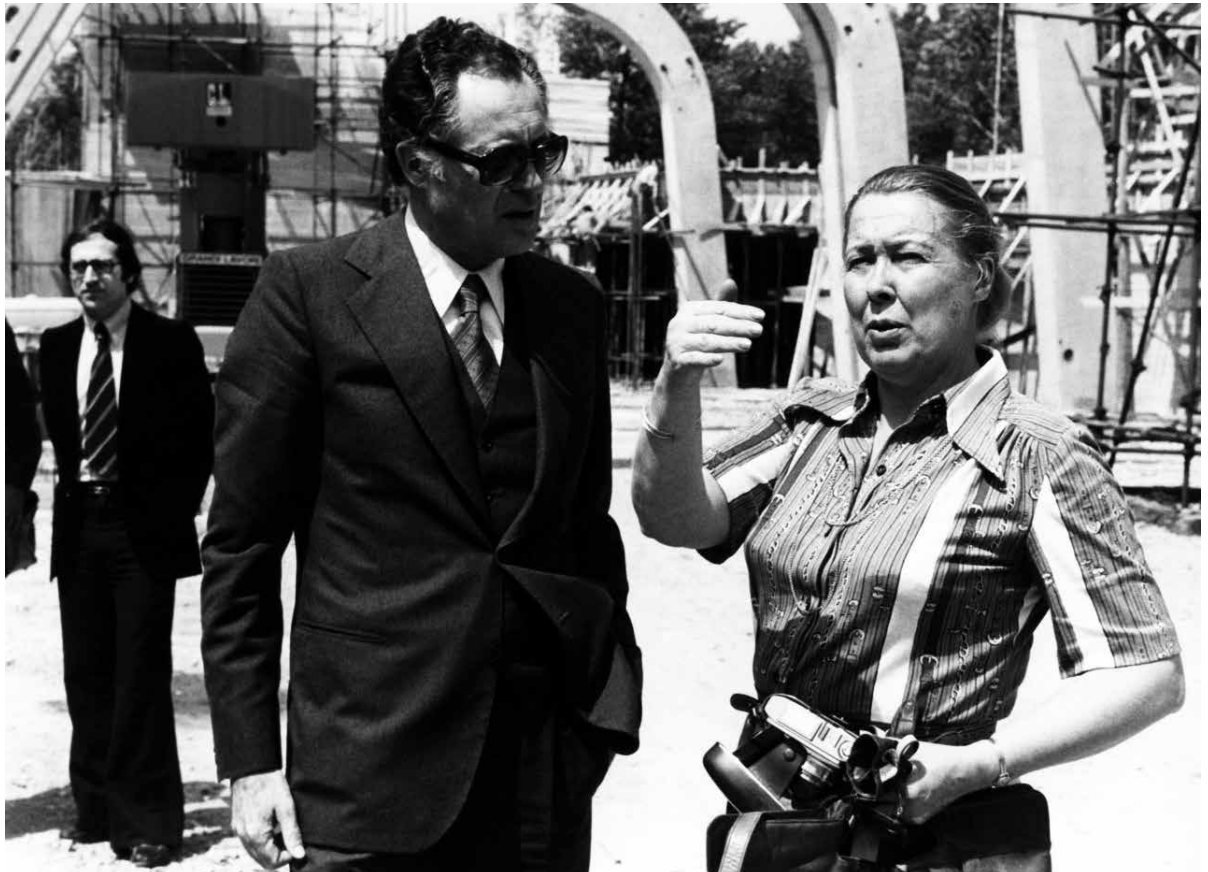
2 Elissa Aalto at the construction site of the Church of St Mary of the Assumption (1966–80) in Riola di Vergato, near Bologna, Italy.
