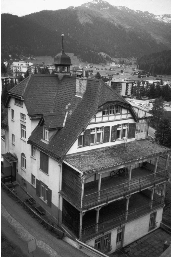
Figure 7: Cast-iron balconies, Haus Caselva (1905), formerly Villa Merula, Davos, Switzerland (author's photograph).
